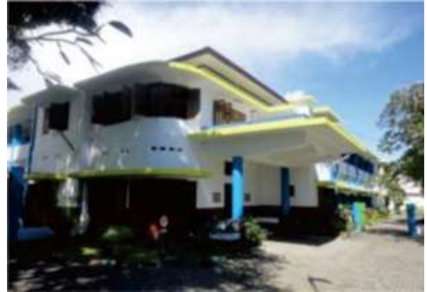
Fig 3. Ratnaningsih Residence, Yogyakarta. Source : Author Documentation, 2017.
